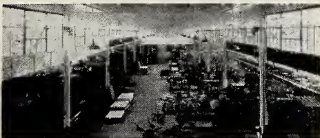
Well-lighted and ventilated interior (Austin No. 2 Standard Building, 90 ft. wide) of the Haddon Press Plant, Camden, N. J.
